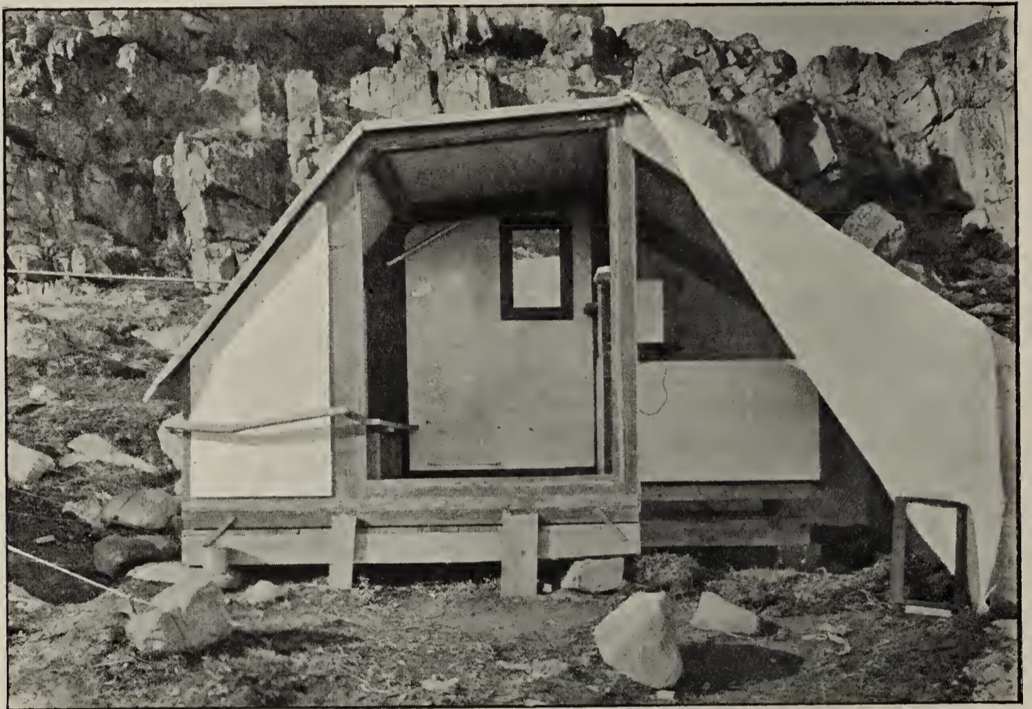
Fig. 7. The respiration chamber in course of erection.
